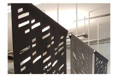
Static track with verticl support rods for lowered panels.
